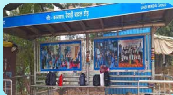
Bus stop renovation, Bawal
